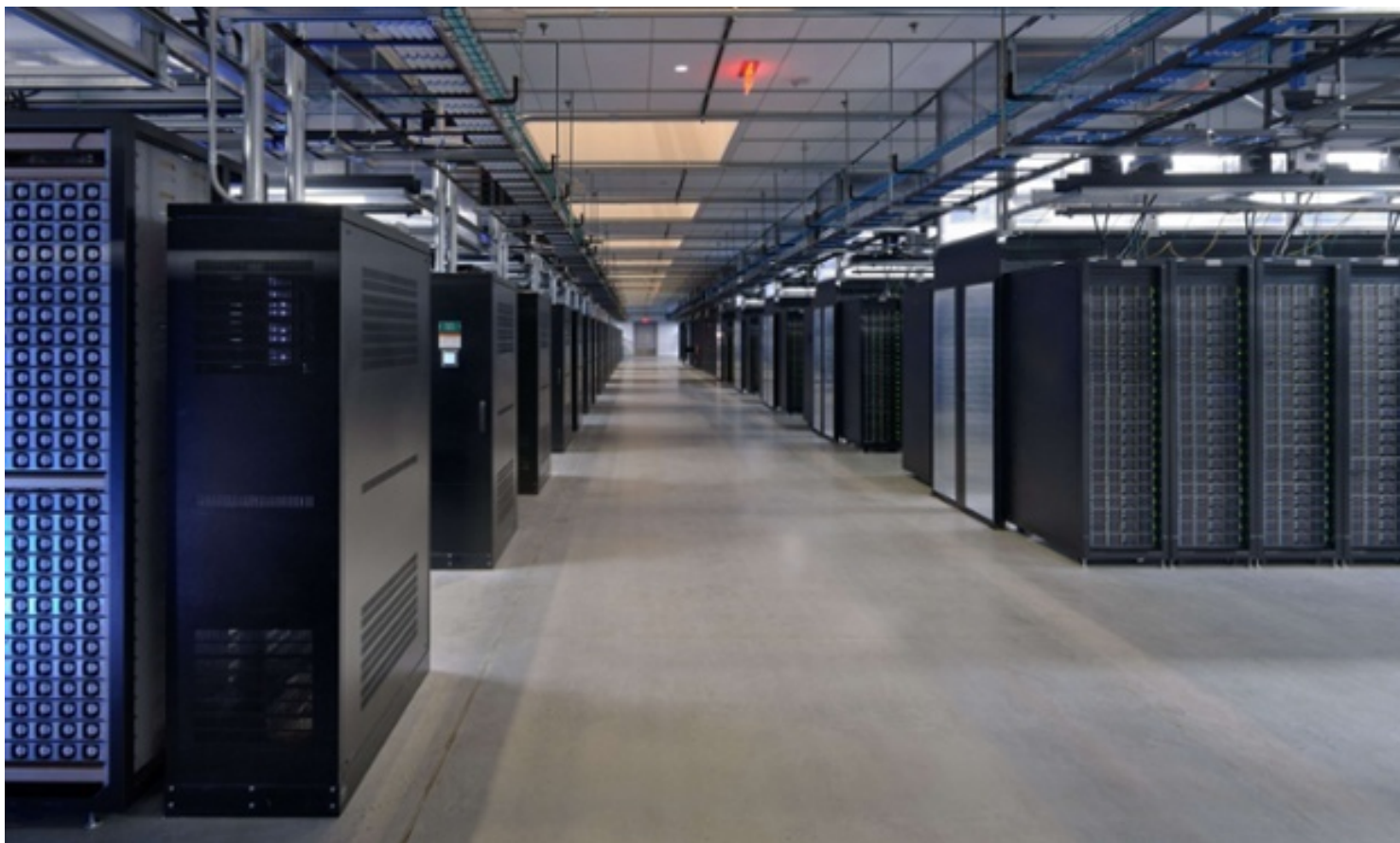
Our secrets in their hands: one of four server rooms at the Facebook data centre in North Carolina. Photograph: Rainier Ehrhardt/Getty
